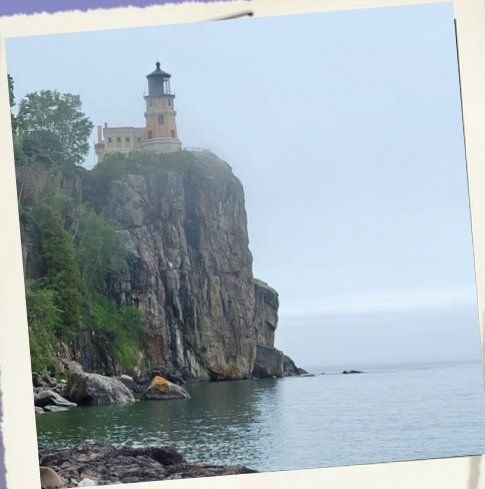
Split Rock Lighthouse
